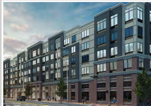
The Crossings at Brick Church Outstanding Project Award
