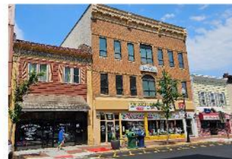
5D Historic facades (adaptive reuse)
